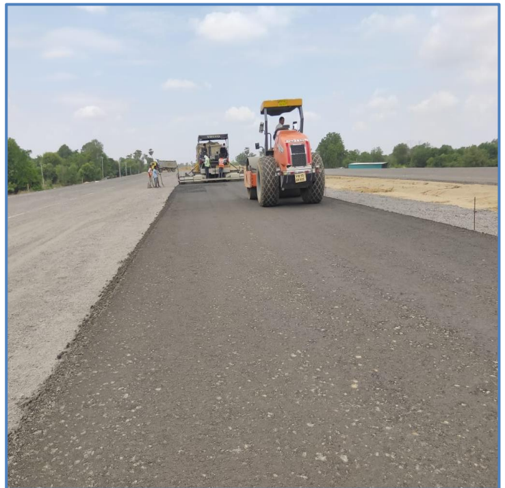
DBM Work In Progress at ch. 362+150 to 362+890
