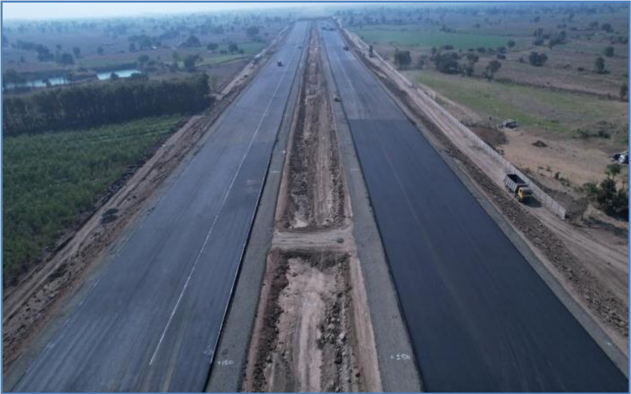
DBM Work In Progress at ch. 362+150 to 362+890
