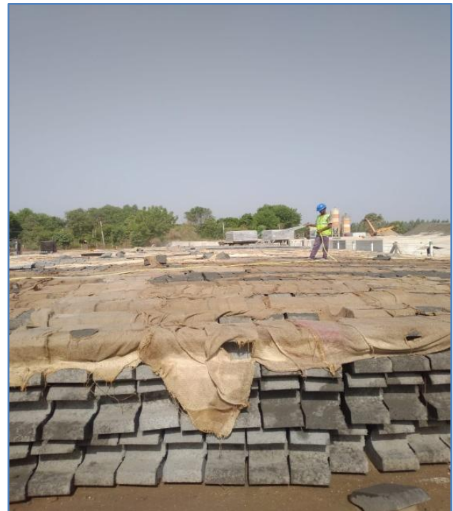
RE block casting and curing at camp casting yard
