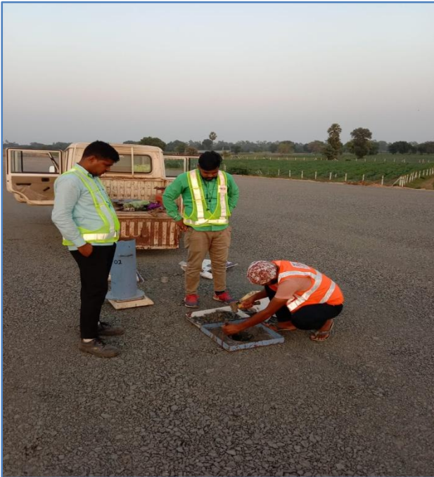
FDD checking at Ch. 351+150 GSB Top
