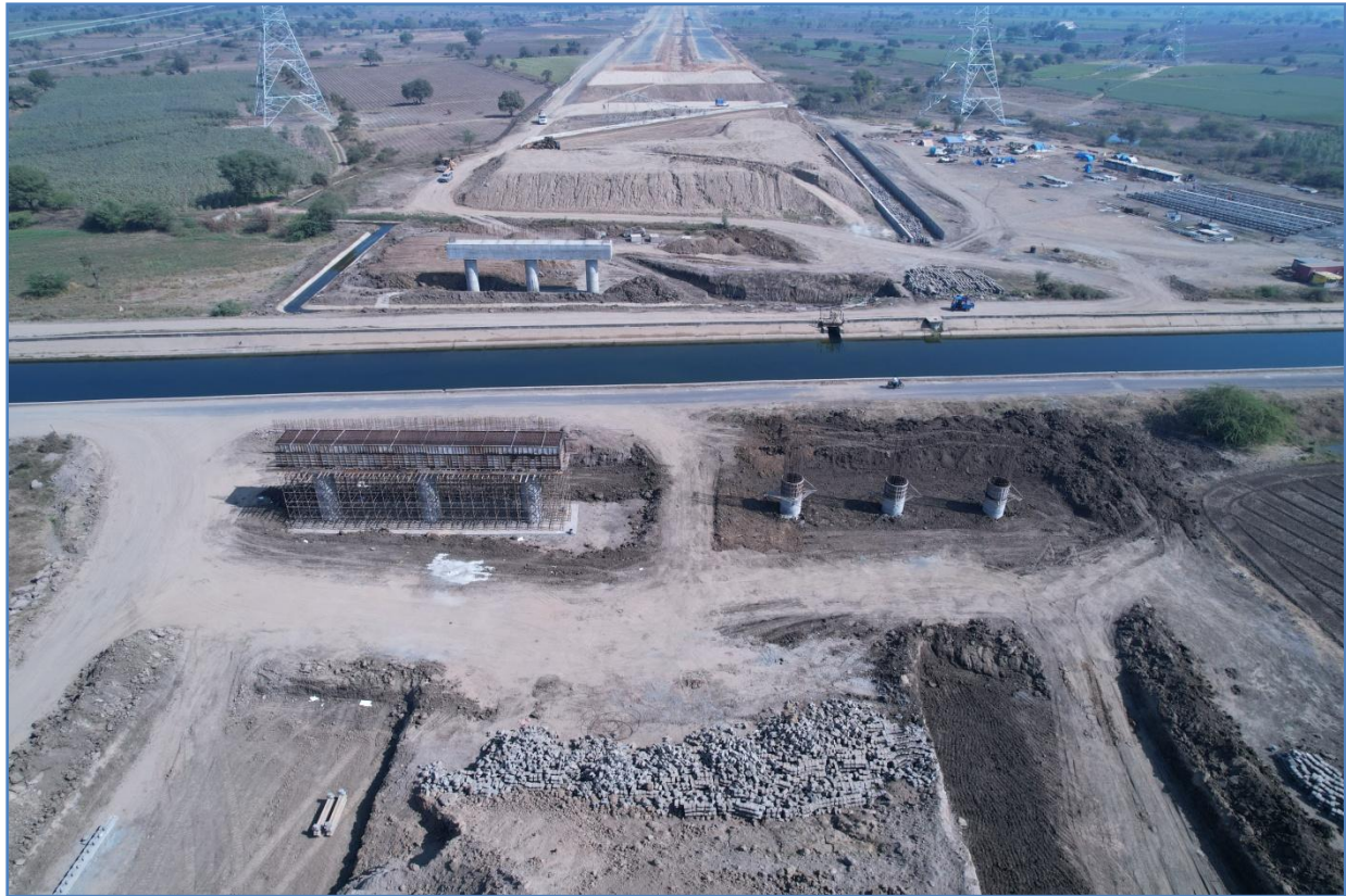
Work In Progress at chainage – 361+839 Major Bridge
