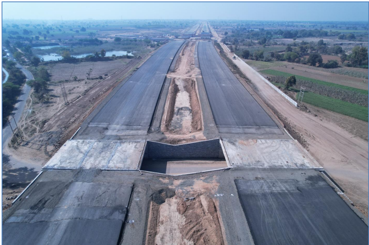
DBM Top Laying at chainage – 359+485 (LVUP Approaches)
