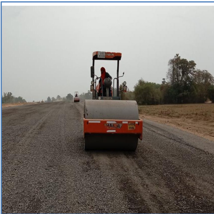
DBM Work In Progress at ch. 362+150 to 362+890
